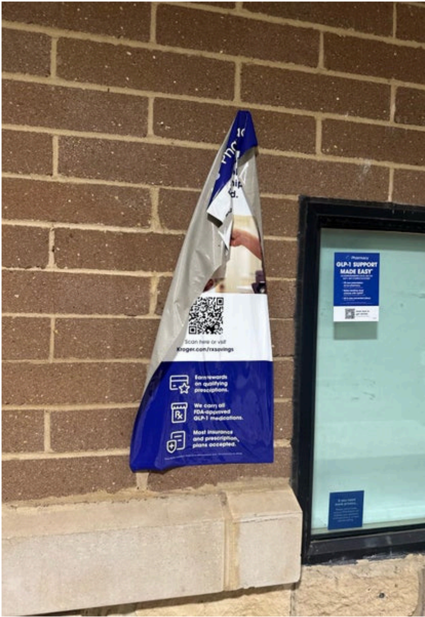
Corners Peeling Remove
