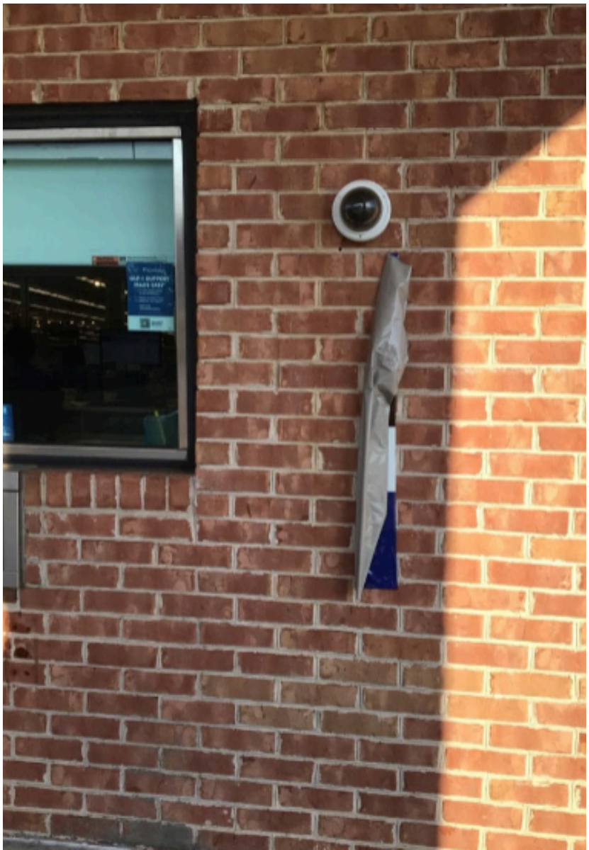
Melting + Peeling Remove
