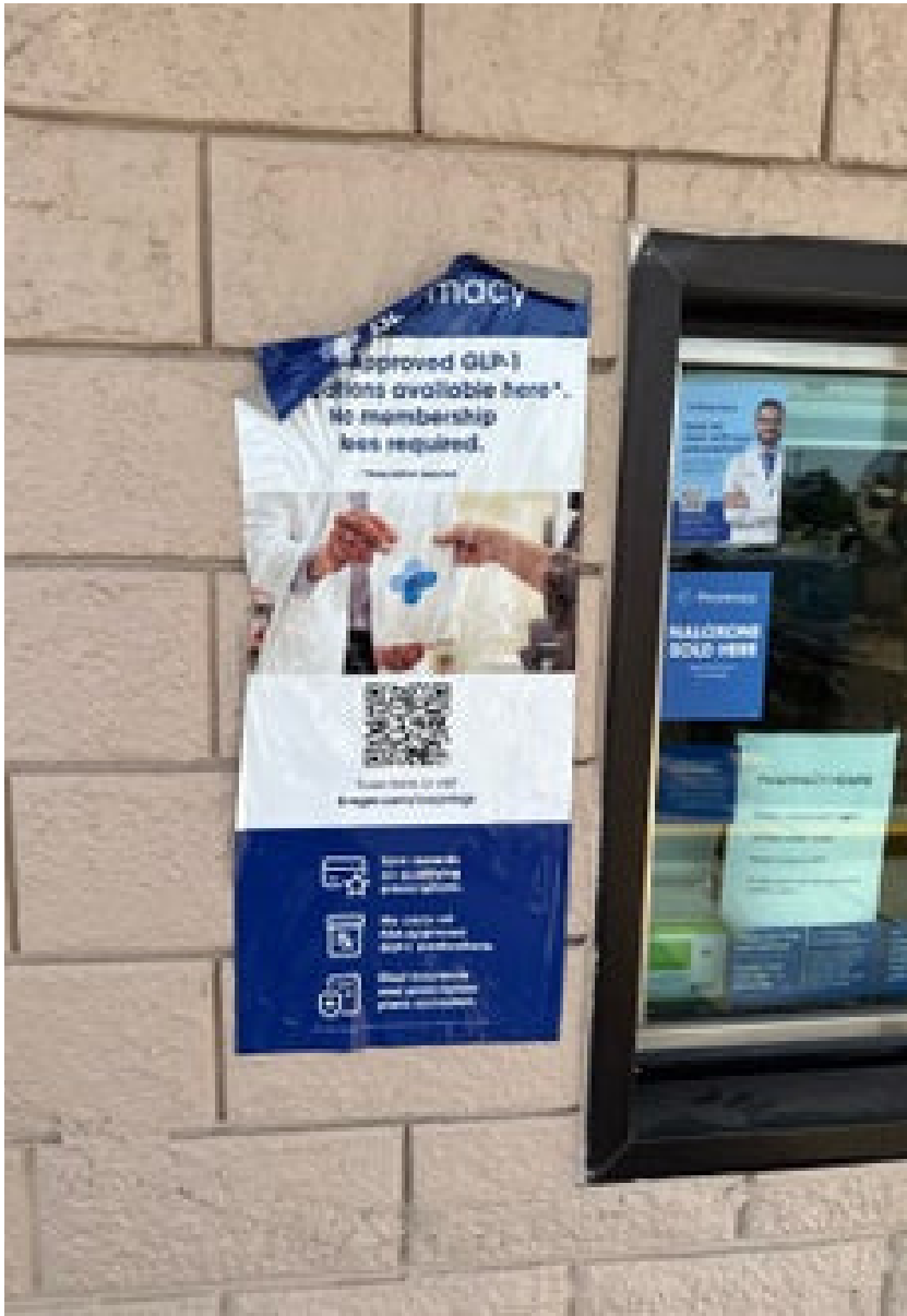
Corners Peeling Remove
